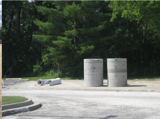
Drainage structures to be used in the bus loop
