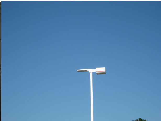
NEW LED on the left and EXISTING on the right
