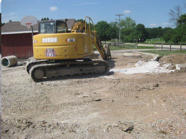
Excavation – MES – East Side
