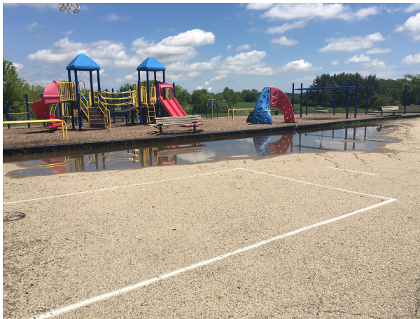
Drainage problem at Millburn Middle School
