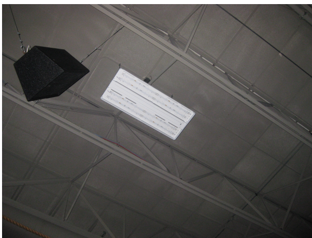
Lighting being installed in the East Gym
