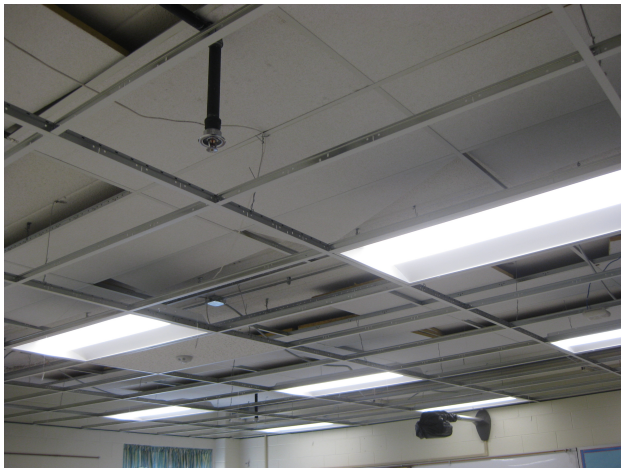
Ceiling grid installed and sprinkler heads relocated
